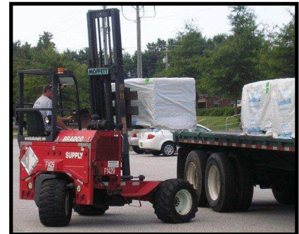
The unloading of the roofing tiles has begun!
